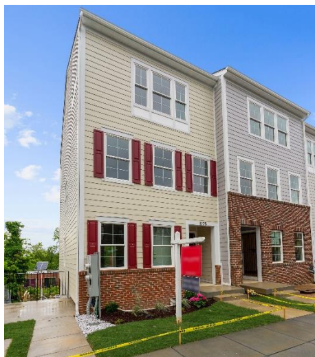
Homeownership development in mixed-townhome and two-over-two configuration in Washington, DC
